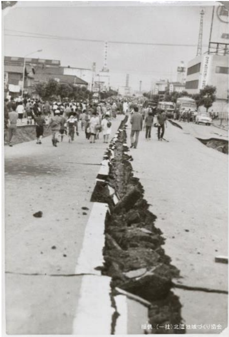
Earthquake crack
